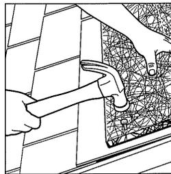
**STEP 3:** Tack one end and unroll entire length of roll to ensure straightness. Multiple pieces simply butt together and tack down. No end plugs are required.
